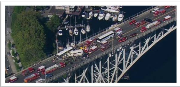
Aerial view of the Aurora Bridge following crash of vehicles
